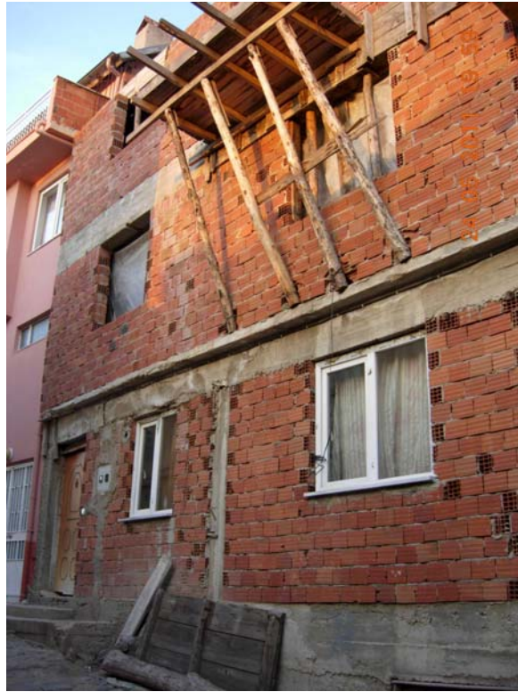
Figure 45: 3 storey building of which infill bricks are being used as a structural load bearing elements, combined with RC beams!!!
