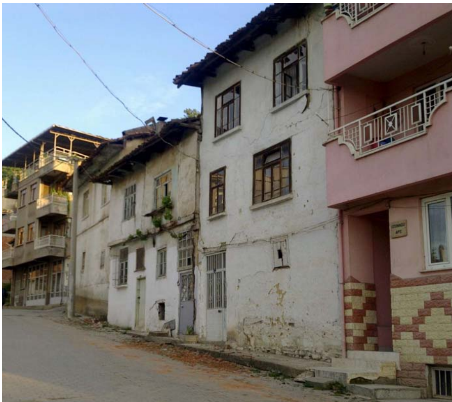
Figure 36: A street view, having adobe and brick masonry buildings - 1
