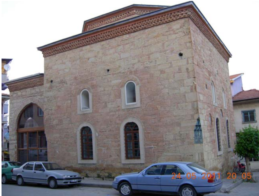
Figure 43: A stone masonry mosque, constructed in the middle of 17th century and recently restored
