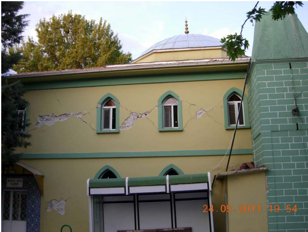
Figure 42: Brick masonry mosque, constructed in 1962
